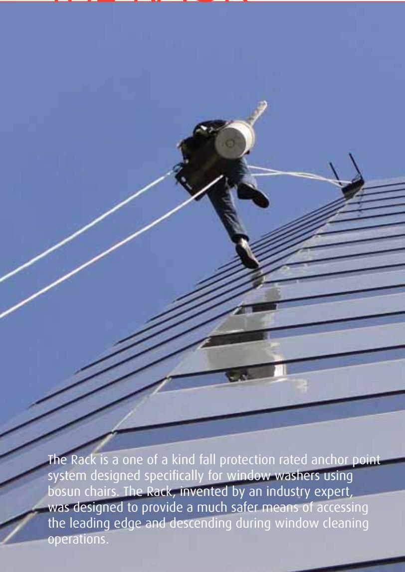
The Rack is a one of a kind fall protection rated anchor point system designed specifically for window washers using bosun chairs. The Rack, invented by an industry expert, was designed to provide a much safer means of accessing the leading edge and descending during window cleaning operations.
