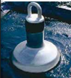
Window Washing Anchor
